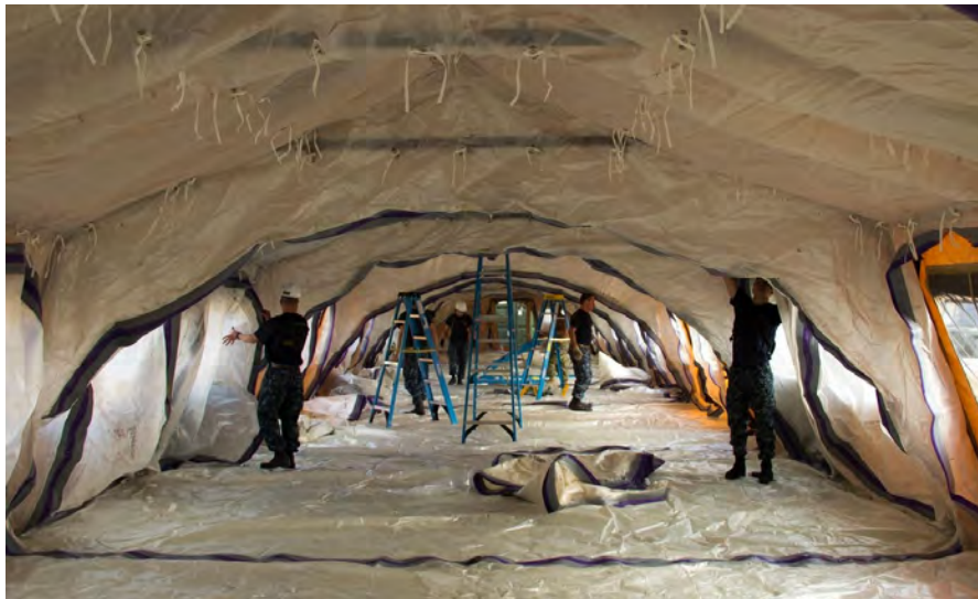
Members of Construction Battalion Maintenance Units 202 and 303 worked closely together installing the Collective Protection inner lining in the Expeditionary Medical Facility during the system evaluation.
